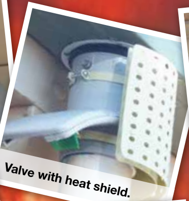
Valve installed in downpipe (in-line).
