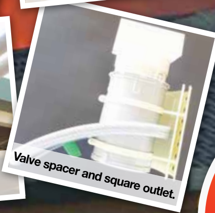
Valve installed in downpipe (in-line).
